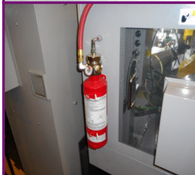
Fire suppression system for Oil
